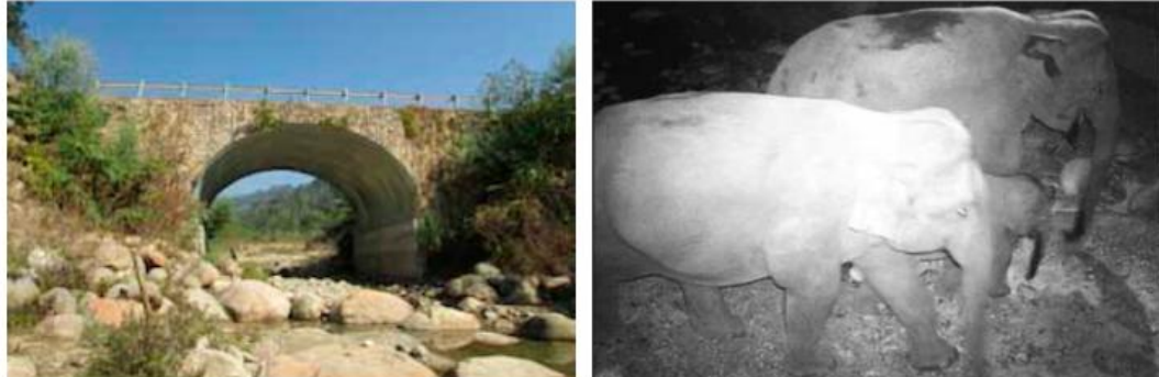
Wildlife underpass constructed and being used by elephants in Samrang, Bhutan.
