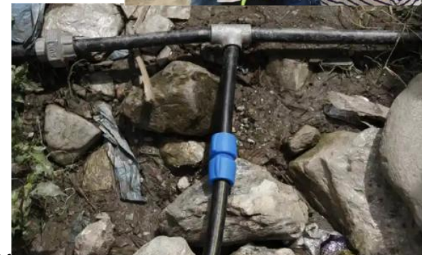
Top Image: Staff from Field Ready use a 3D printer to create a custom pipe fitting in Nepal following the 2015 earthquake. Bottom Image: Blue custom fitting produced using a 3D printer. Image source: Jones, Sam. 2015. When Disasters Strike, It's Time to Fly In the 3D Printers. The Guardian. December 30.
