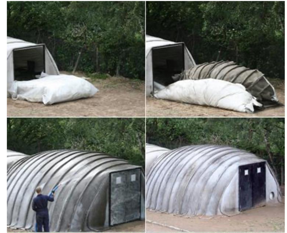
Image: Concrete Canvas ® shelter in various stages of installation Source: Flood Control International, 2019.
