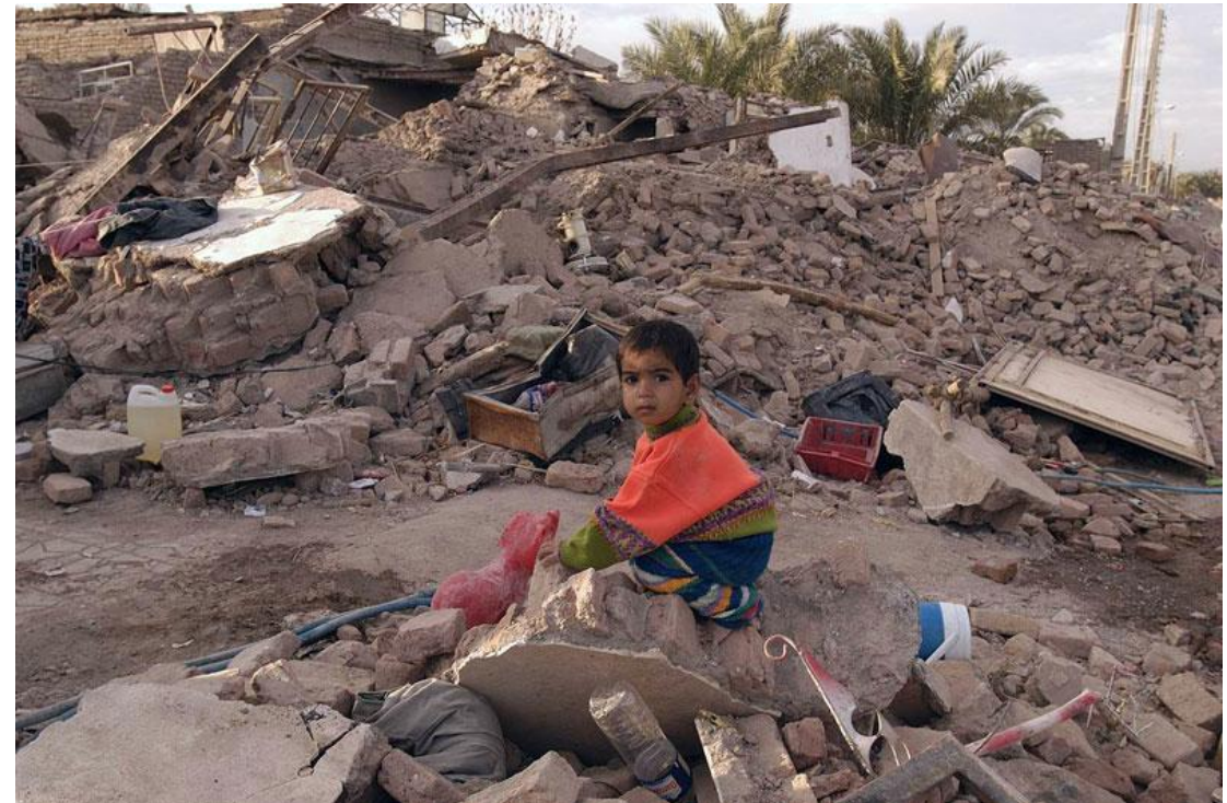
Image: Traditional earth-brick homes that are highly vulnerable to seismic risk were ultimately to blame for the majority of deaths that occurred during the Bam Earthquake in 2004. Image credit: Shehzad Noorani, UNICEF Iran.
